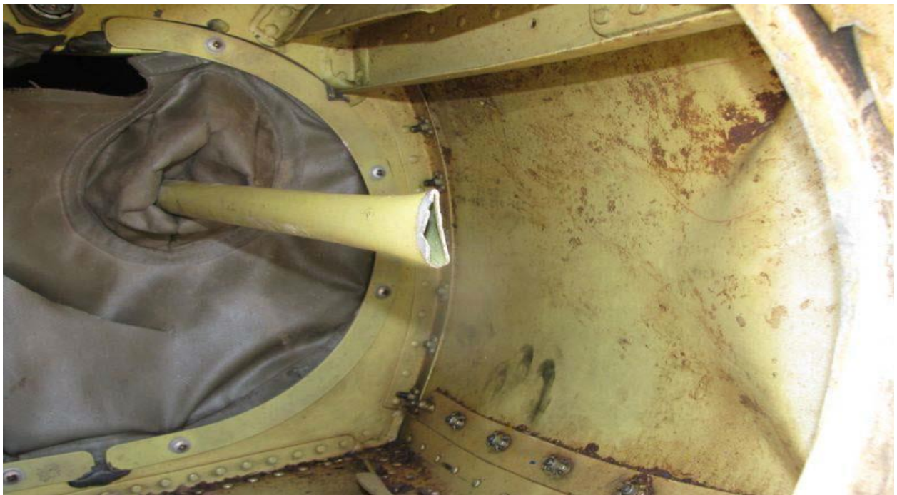
Picture14 Overload fracture of long tail rotor control tube near aft fuselage tailboom attach point
