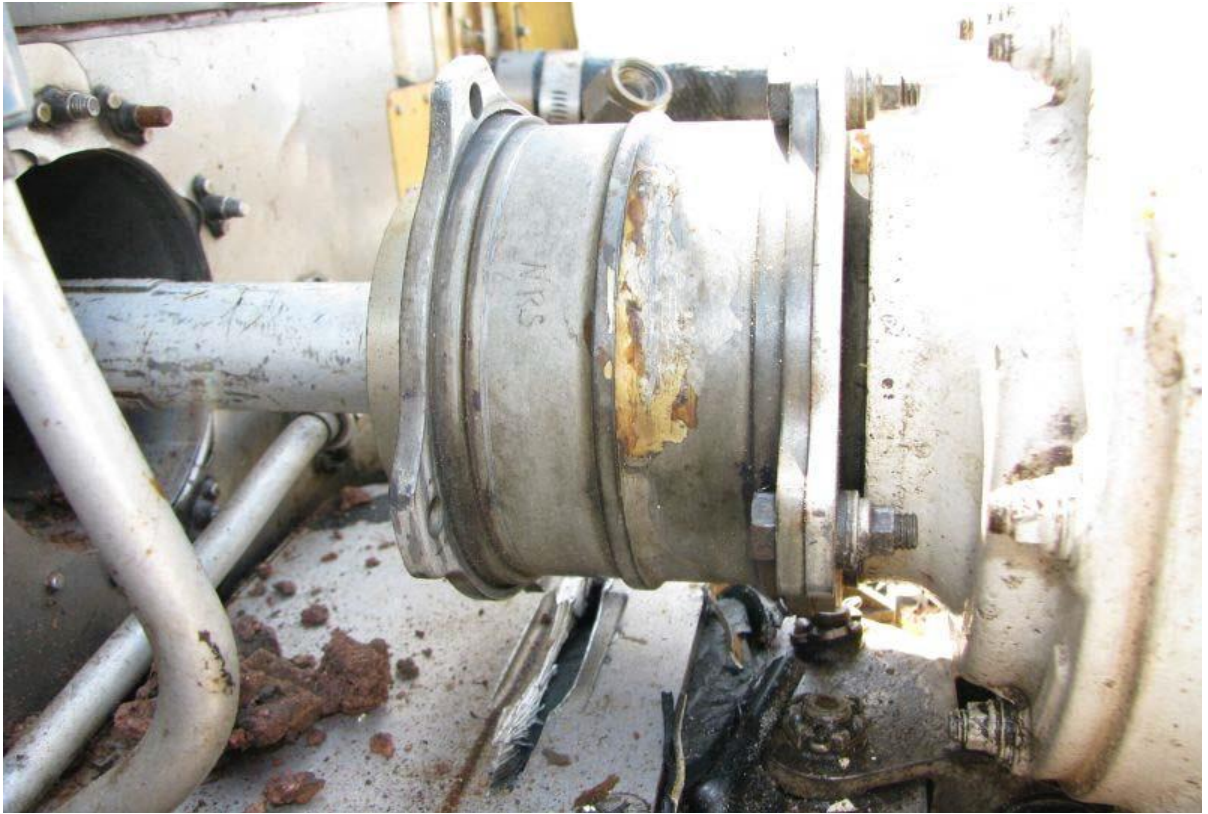
Picture 3 Forward outer main driveshaft coupling with no temp dot arrays installed
